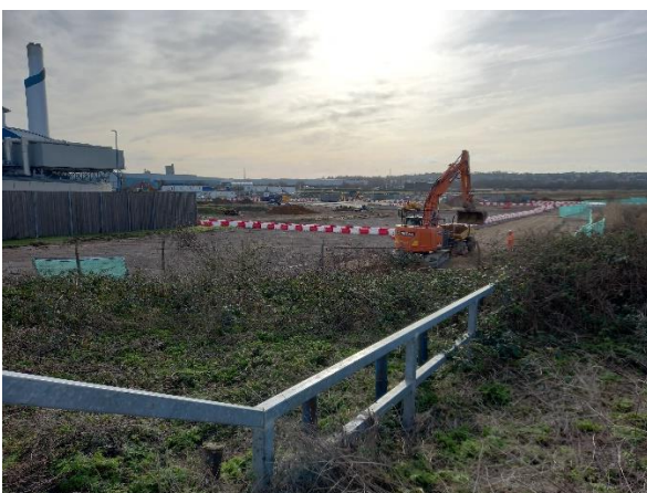
Construction zone within the Riverside 1.
